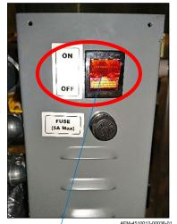
Boiler Controller Power Switch (Off)
