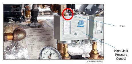
**NOTE:** If the pressure exceeds 85 PSIG, a Pressure Tab on the top of the High Limit Pressure Control pops out and needs to be reset by pushing it down.
