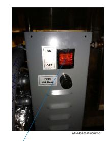
Boiler Controller Power Switch (On)
