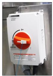
/ AFM-4510012-00053-01 System Main Power Switch (Off)
