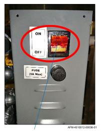
Boiler Controller Power Switch (Off)
